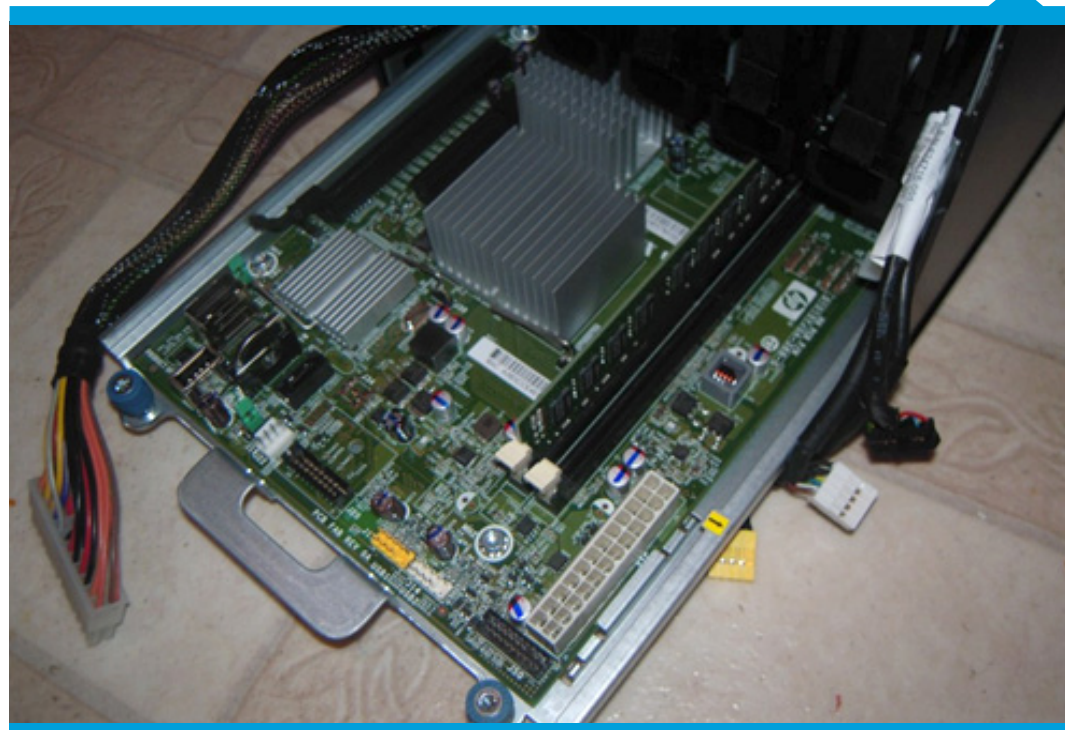
N40L Motherboard Tray, partially removed
